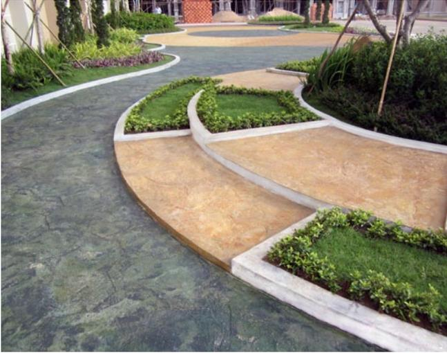
**Exterior Decorative Concrete Overlays** are engineered to be a surface repair or an aesthetic finish that can be applied to new or existing concrete surfaces. The finished application is actually stronger than concrete and can withstand vehicular traffic and harsh temperatures (extreme hot or cold).
